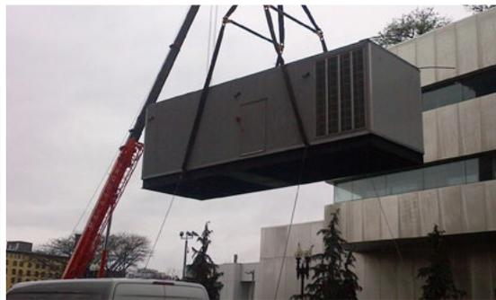
The first of the 4 emergency generators is lifted onto the lower roof. The generators' location was changed from B2 as part of the Bank's resiliency planning, to mitigate the impact of natural disasters and a potential rise in sea level.
